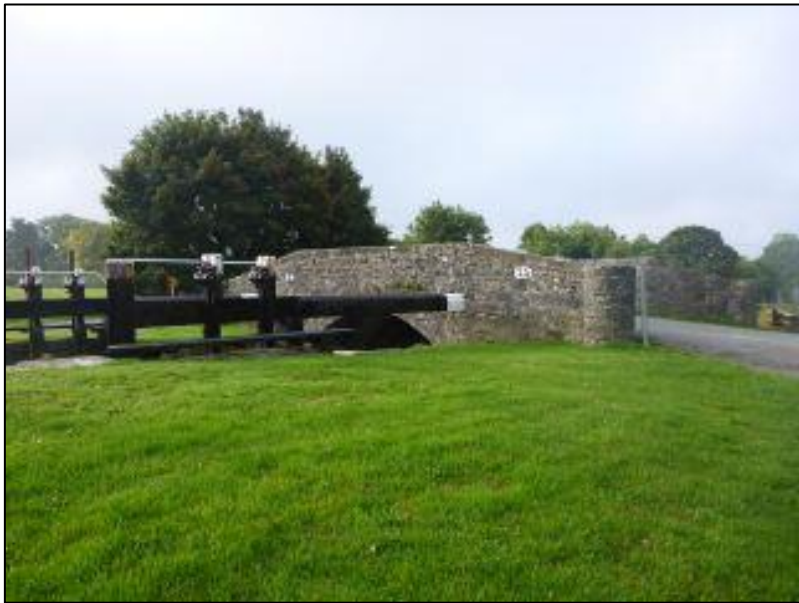
Illus. 14. 65 Glenaree Bridge and Lock 22 Grand Canal Barrow Line (RPS B17-16)
