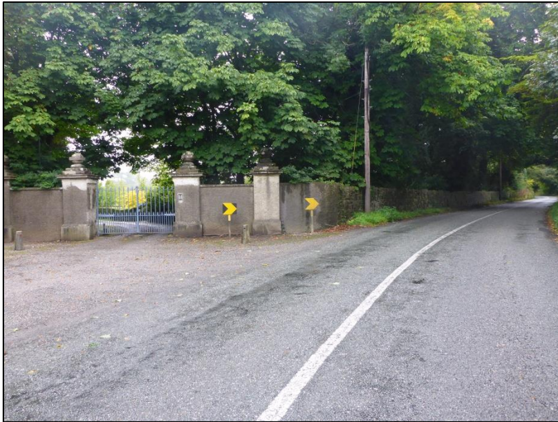
Illus. 14. 33 Entrance Gates into the southernmost entrance to Williamstown House (RPS B03-06)
