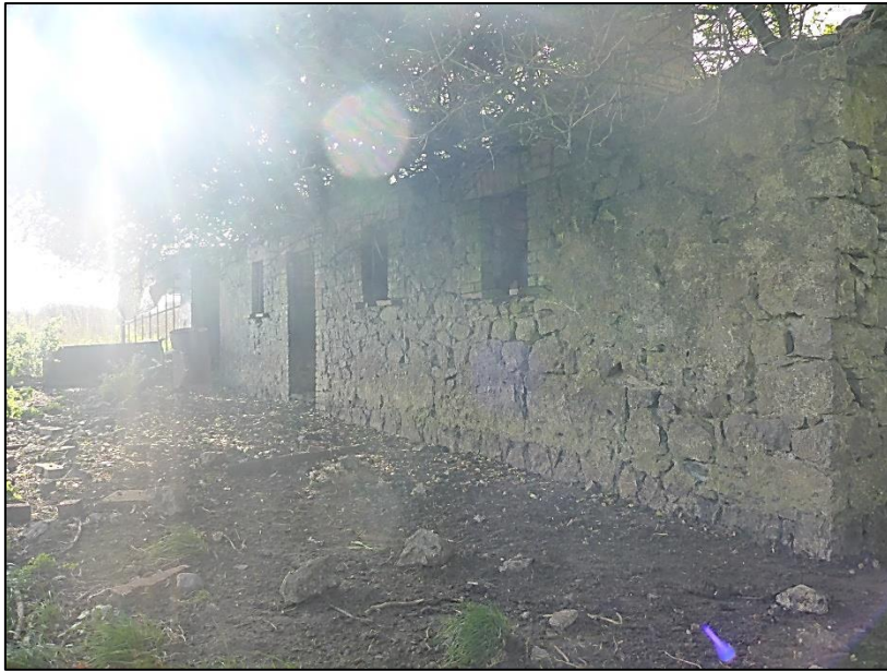
Illus. 14. 46 Roofless ruin of a vernacular structure in Hortland
