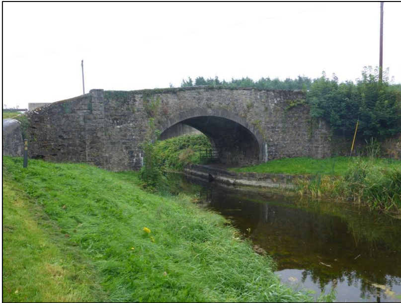
Illus. 14. 12 Moyvally Canal Bridge
