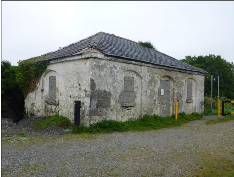
Illus. 14. 10 Canal workers house (RPS MH047-204)
