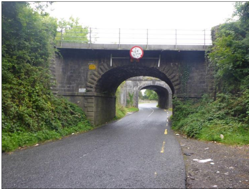
Illus. 14. 11 The Railway Bridge (foreground, RPS MH047-202) and the canal aqueduct (RPS MH047-201)
