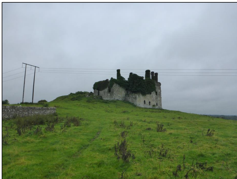
Illus. 14. 74 Fortified house/ castle KD008-00102-03) on the northern shoulder of Carbury Hill
